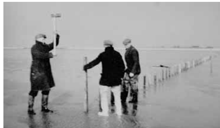
EA photo showing local people building their own flood defences on the Humber in the 1950's, clearly demonstrating their understanding of local coastal processes.
